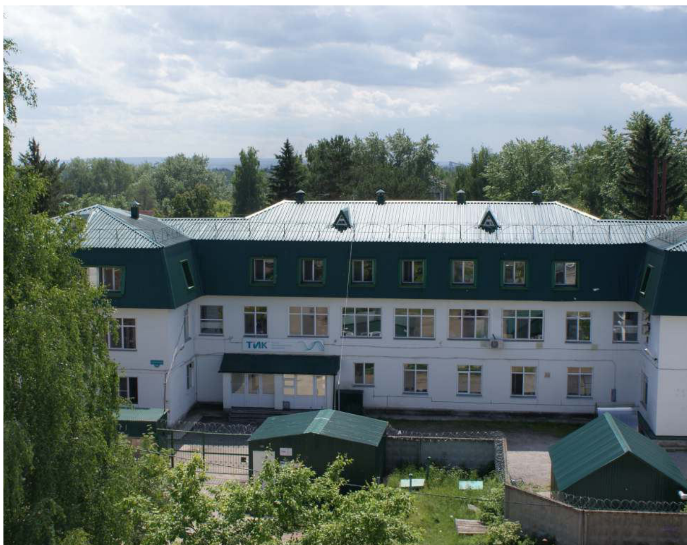
Building of RPE «TIK», production area TIK-1
