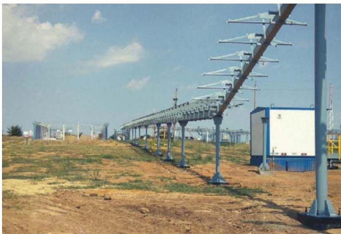
Construction of cable overpasses at the Customer's facility
